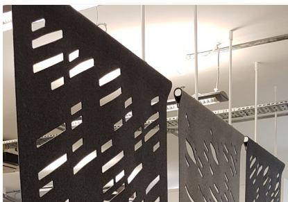
Static track with vertical support rods for lowered panels.
